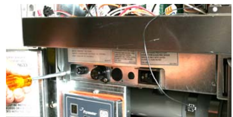
Figure 2: Remove access panel under computer.
